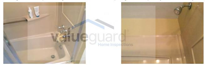
The diverter was noted to not be fully functional. All water should be directed to the shower when the diverter is engaged. Recommend necessary repair/replacement to restore proper function.
