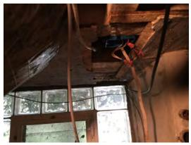
Abandoned wiring was noted. This wiring should be removed or properly terminated for improved safety.
