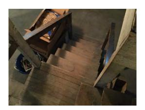
Absent handrail(s) observed. Graspable handrail(s) are advised at stairs which have 4 or more risers for safety.
