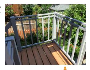
Joists were noted to be out of plumb and not flush with floor boards. Repairs by a qualified contractor are recommended.
