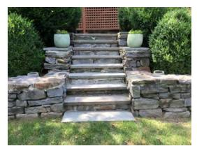
Absent handrail(s) observed. Graspable handrail(s) are advised at stairs which have 4 or more risers for safety.
