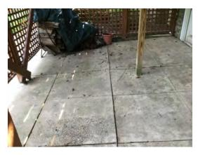
Cracking in the patio observed. Sealing the cracks is advised to prevent additional cracking and damage.
