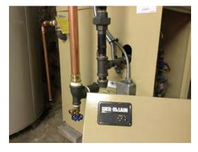
Venting of exhaust gas is accomplished without the aid of mechanical fans or boosters. This is basically a vertical system. The temperature difference between the exhaust gas and the atmosphere creates a draft that exhausts gasses to the atmosphere.
