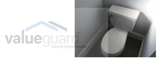
Toilet was observed to "run-on" after flushing. "Run-on" is typically the result of a damaged or misadjusted fill mechanism. Recommend necessary corrective action and confirmation of proper function.
