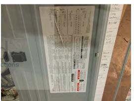
The panel was partially labeled. Recommend properly labeling the panel.
